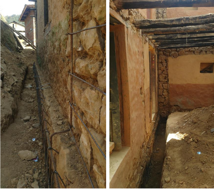
Ring Concrete Bands at Plinth Level, inside and outside views
