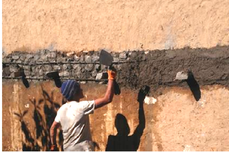
Ring Concrete Bands at Floor Level, outside view
