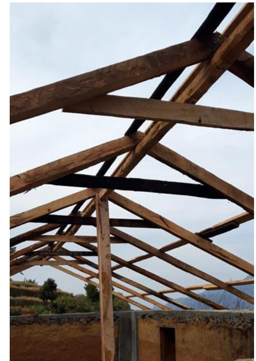
Roof retrofitted with tying by collar beams
