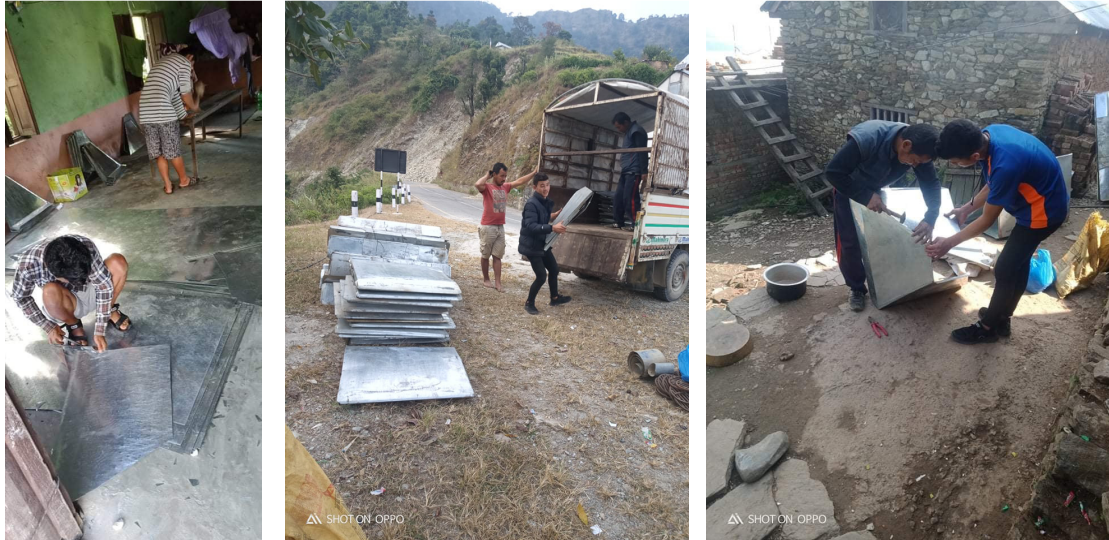
Manufacture, transportation and assembling of the metal parts of a smokeless kitchen: the hood and the chimney.
