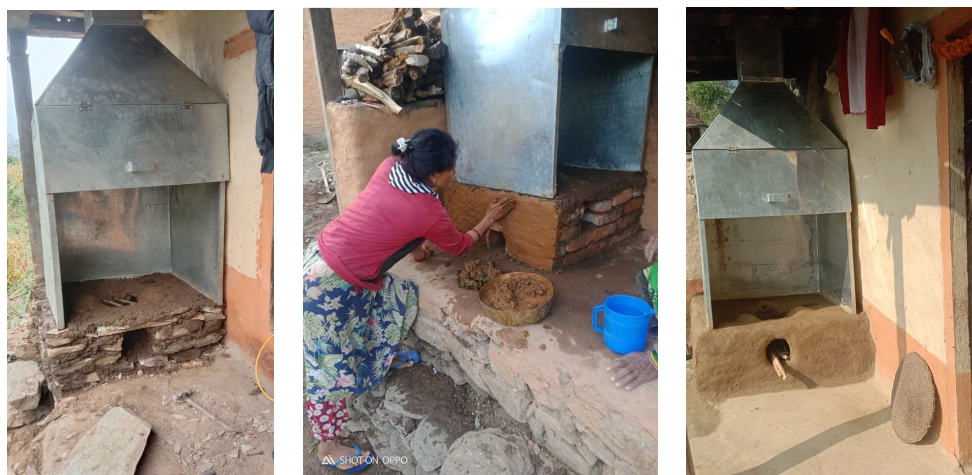
Improved Cooking Stove (ICS) made with mud and stones, seen in three different stages: without the final layer of mud finishing, woman applying the final mud layer and the final result.
