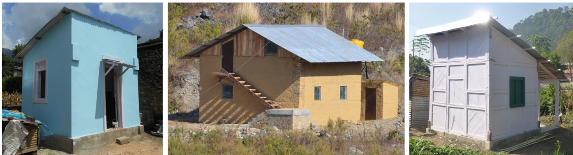
From left to right: "confined block", "stone and mud" and "wood" prototypes respectively.
