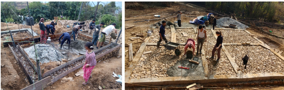
Foundations of the new houses in Supin.
