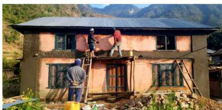
The retrofitted houses in Supin almost finished, lacking only all the wooden diagonals.
