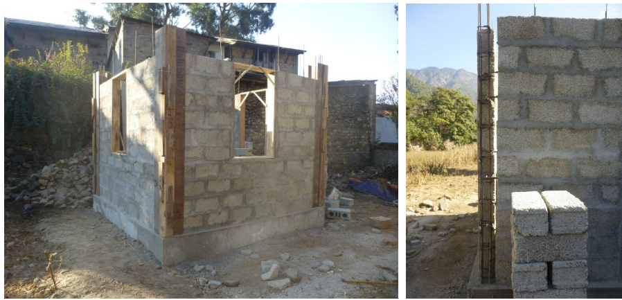
Concrete Block Prototype, minimum house for Santamaia Didi, caretaker at Balmandir Children's Home.
