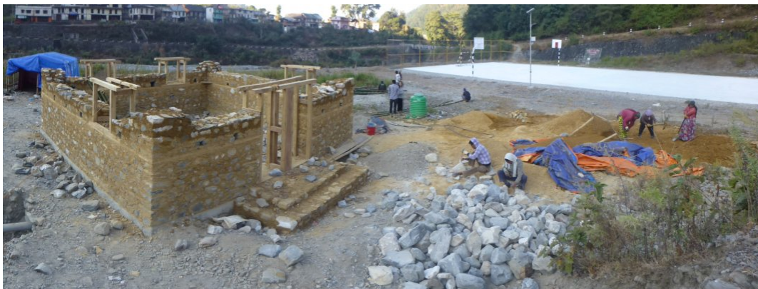
Stone and Mud Prototype, future building for changing rooms and other facilities for the sports court.
