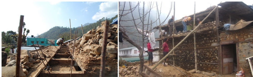
Retrofitting Prototype, stone and mud. Repaired and retrofitted house, Pradhan family.
